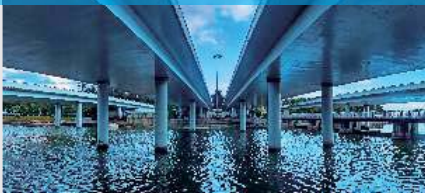
Smart Treatment for Water
